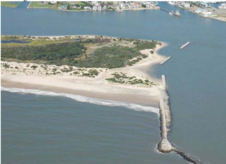
Figure 7: Erosion noted behind the seawalls at the north end of Assateague Island on 8/29/11. Photo by Assateague Coastkeeper.
